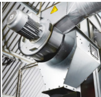
Fan unit with motor and cleaning unit
